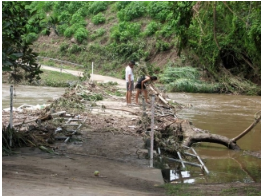
Figure 2.7 – Debris caught on bridge rails
