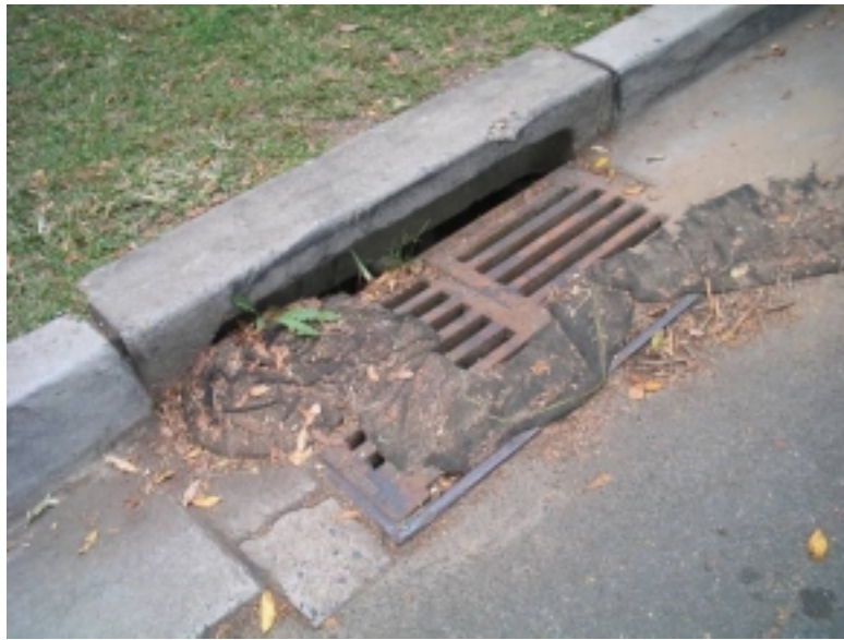
Figure 2.11: Builders material and sediment controls can block culverts
