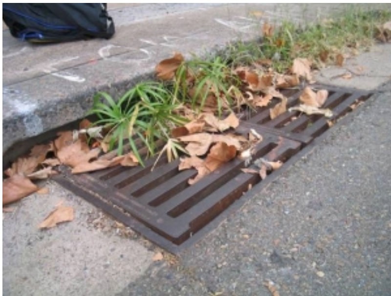
Figure 2.12: Vegetation growing in inlet indicates poor maintenance
