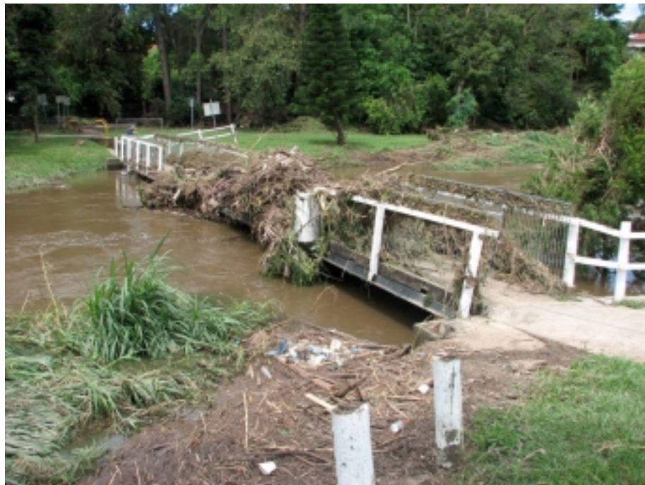
Figure 2.13: Guardrails on a bridge can collect debris
