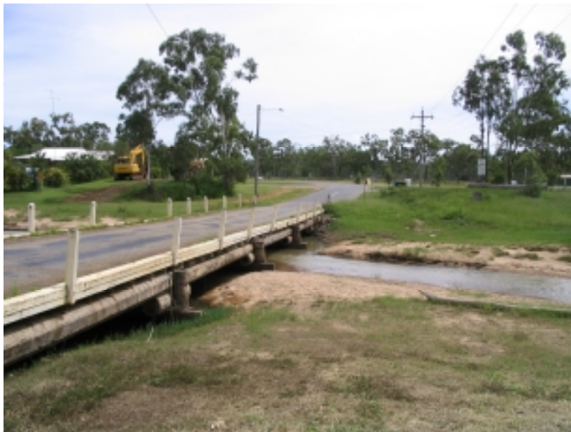
Figure 2.17 – Sedimentation under a bridge
