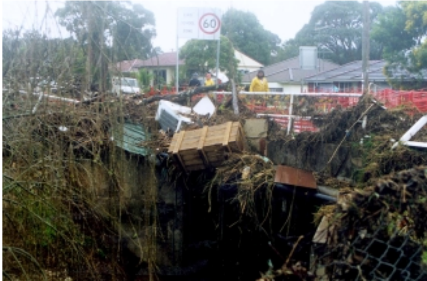
Figure 2.3 – Large Floating Debris Collection
