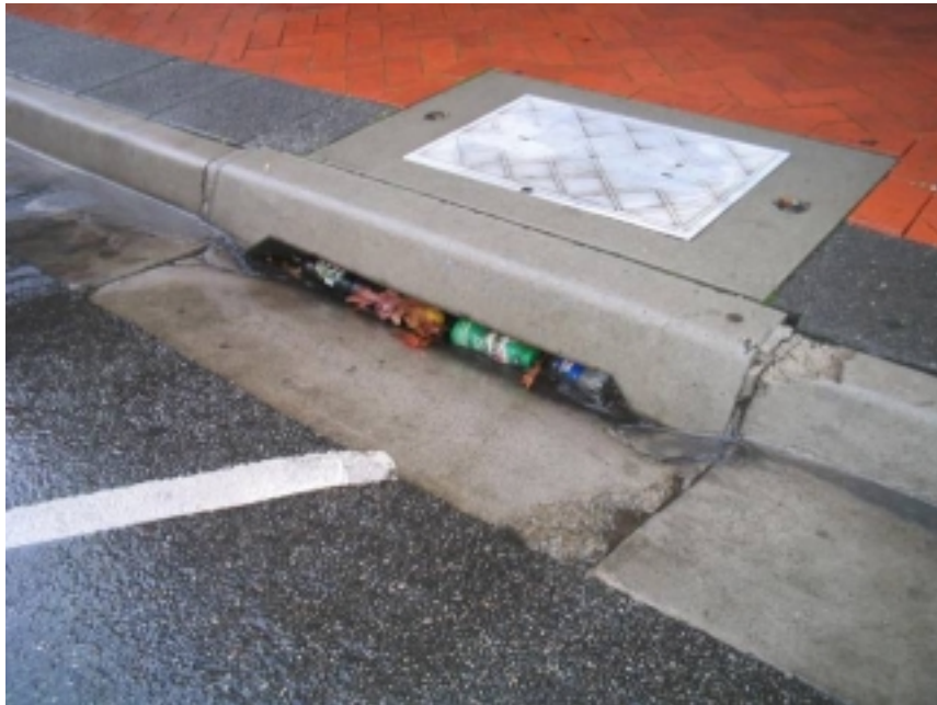
Figure 2.10: Litter in an inlet
