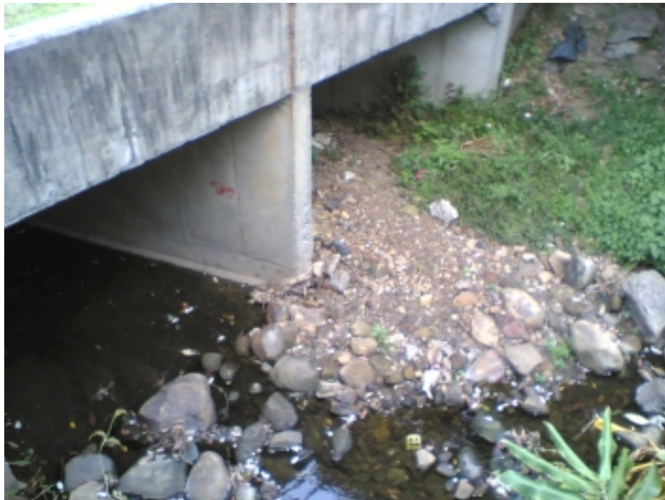
Figure 2.15 – Example of Partial Inlet and Barrel Blockage
