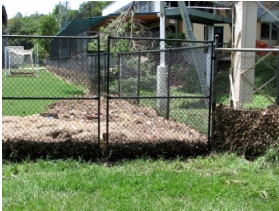
Figure 2.14: Fences collect debris and block overland flow paths
