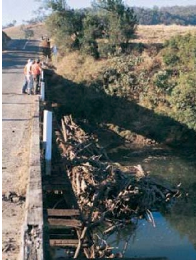
Figure 2.16 – Floating debris on a bridge
