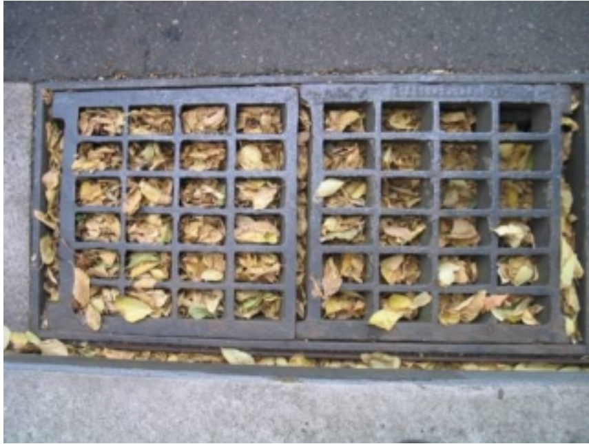
Figure 2.9: Leaves can completely block inlets
