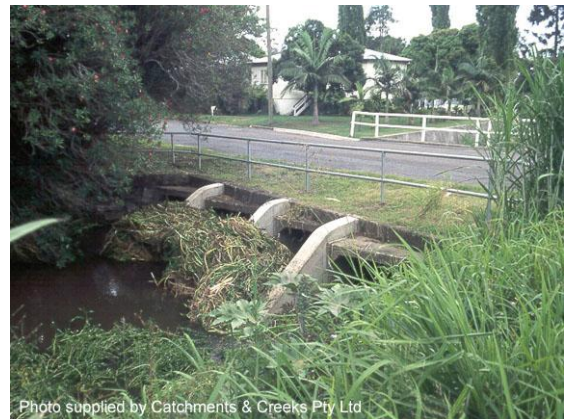
Photo 31: Post flood collection of debris on top of deflector walls
