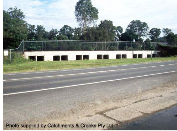
Photo 29: Floodplain culvert
