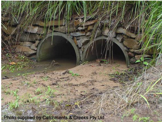
Photo 4: Sediment blockage of stormwater pipes
