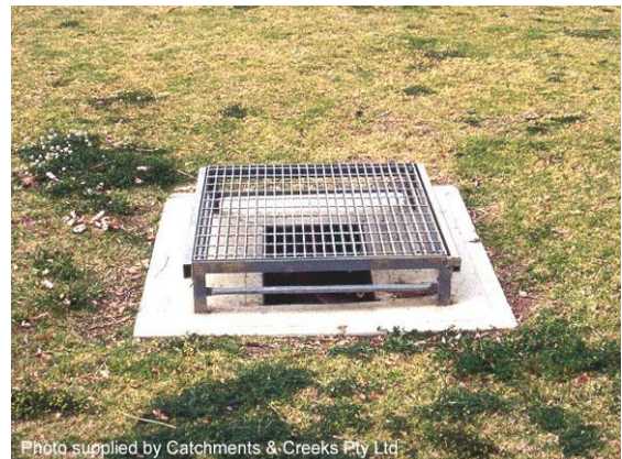
Photo 25: Horizontal screened field inlet with scour control concrete lip
