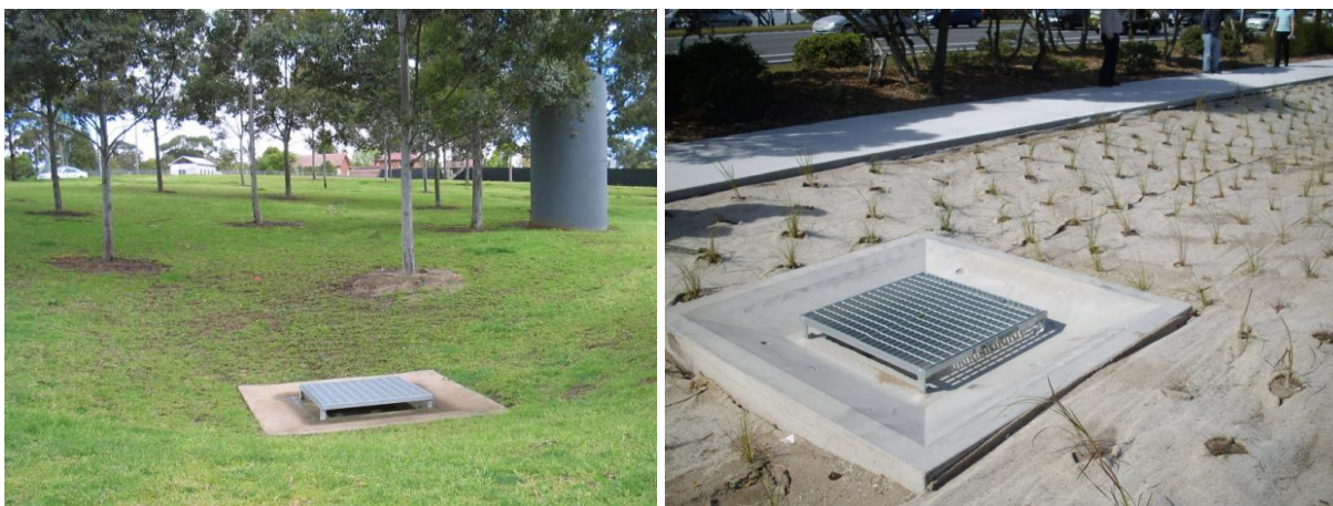
Photo 19A 'Letter Box' Pits in an Open Area and a Bioretention System
