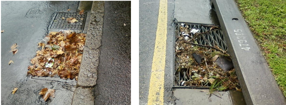
Photo 17: Examples of Grated Pit Blockages, Sydney
