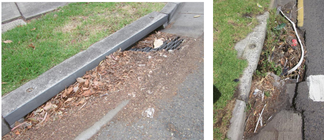
Photo 18: Examples of Kerb Inlet Pit Blockages, Sydney
