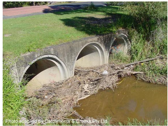
Photo supplied by Catchments & Creeks Pty Ltd Photo 3: Debris blockage of culvert inlet
