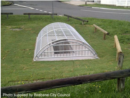
Photo 22: Combined debris and safety screen surrounding a field inlet
