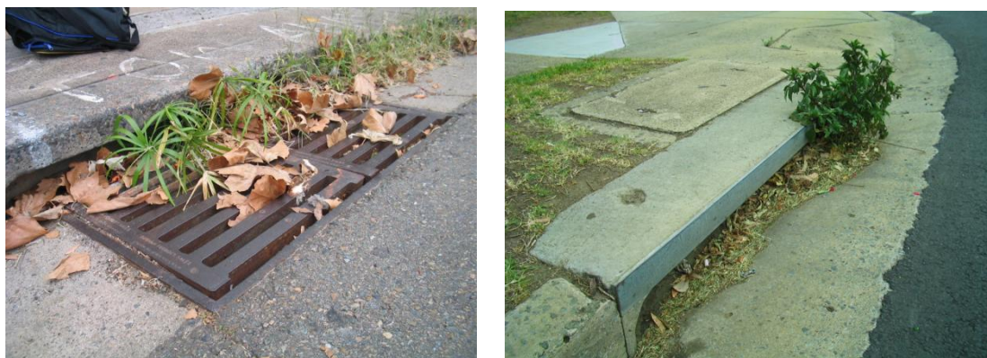
Photo 21: Poor Pit Maintenance
