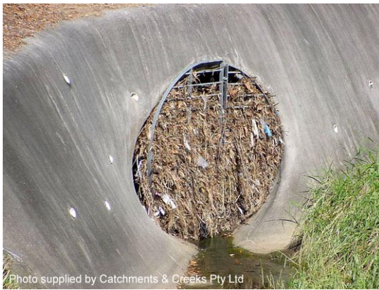
Photo supplied by Catchments & Creeks Pty Ltd Photo 2: Debris blockage of culvert outlet
