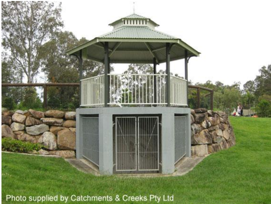
Photo 26: Detention basin outlet chamber
