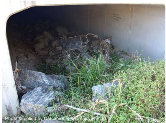
Photo 5: Boulder sourced from an upstream rock chute, now deposited in a culvert
