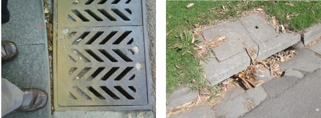
Photo 16: Examples of Pit Blockages, Sydney and Melbourne
