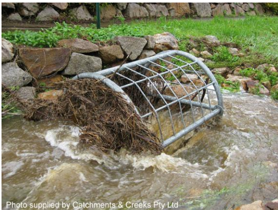
Photo 24: Dome inlet screen with minor blockage
