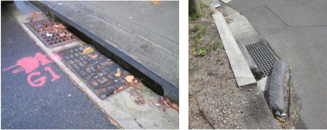
Photo 19: Deliberate Blockages for Sediment and Erosion Control
