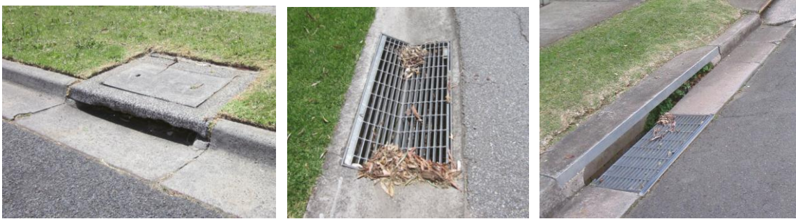
Kerb Inlet, Grate and Combination Inlets
