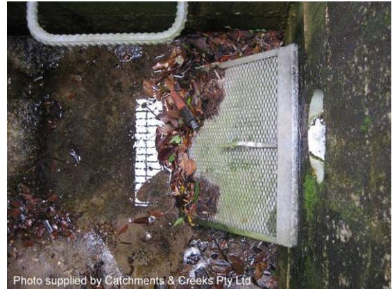
Photo 27: Outlet screen of an on-site detention pit viewed from the screened surface inlet (visible in reflection)
