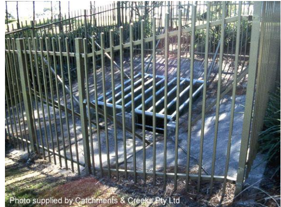
Photo 23: Safety screen surrounding screened detention basin outlet
