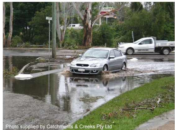
Photo 11: Temporary blockage of kerb inlet causing road flooding
