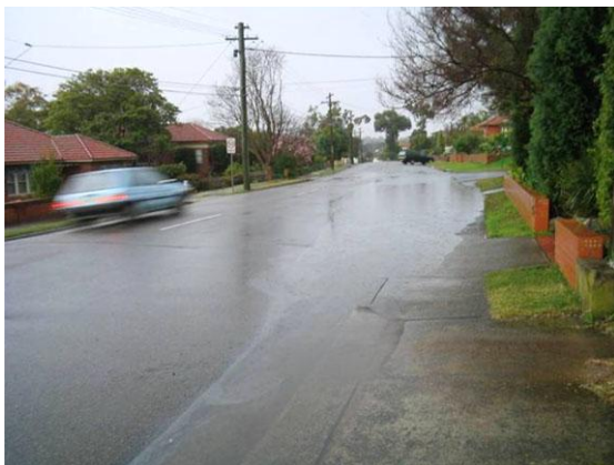
Photo 10: Ponding on street caused by blocked inlet pit (G O'Loughlin)
