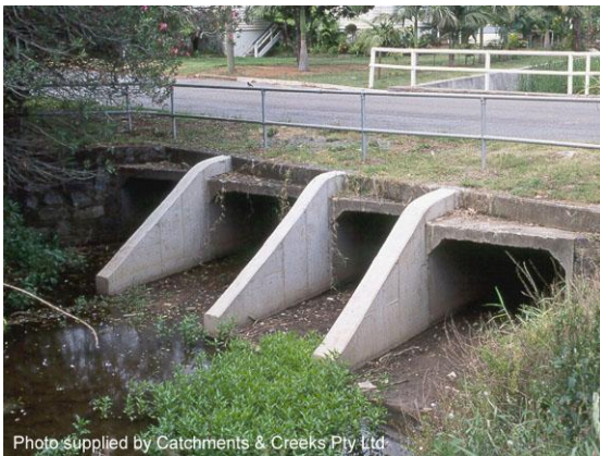
Photo 30: Debris deflector walls
