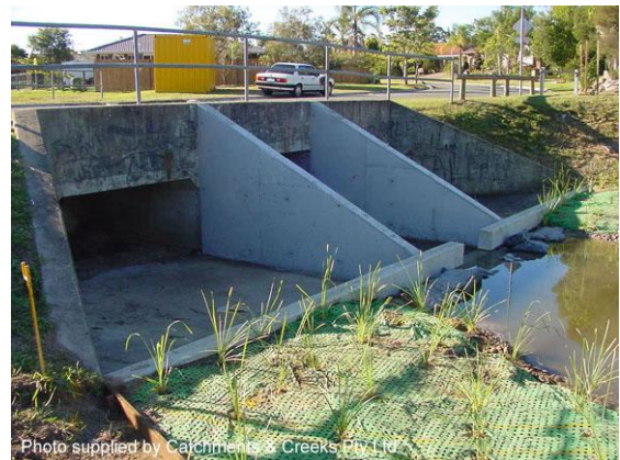
Photo 33: Debris deflector walls and sediment training wall added to existing culvert
