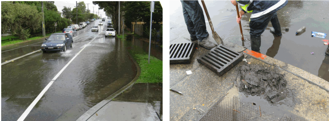
Photo 20: Pipe Blockage Incident, Penshurst, June 2009
