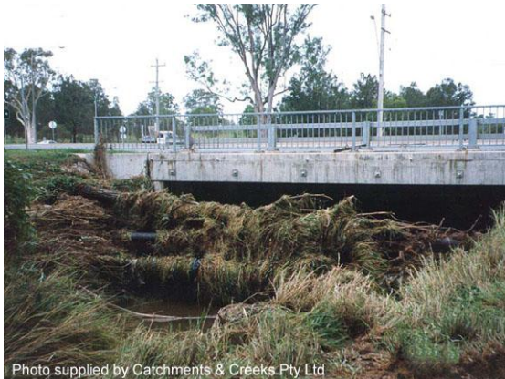
Photo 12: Debris collected around exposed pipes
